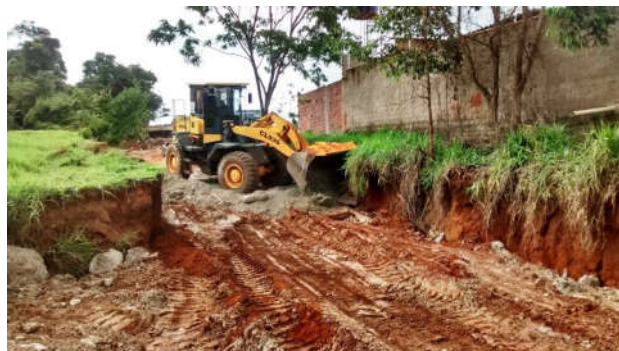
Figure 6. Reshaping the gully
