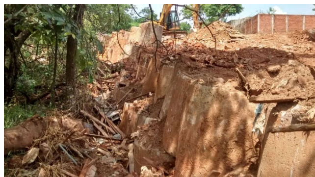
Figure 4. Palisade of water and sewage shackles installed in gullies
