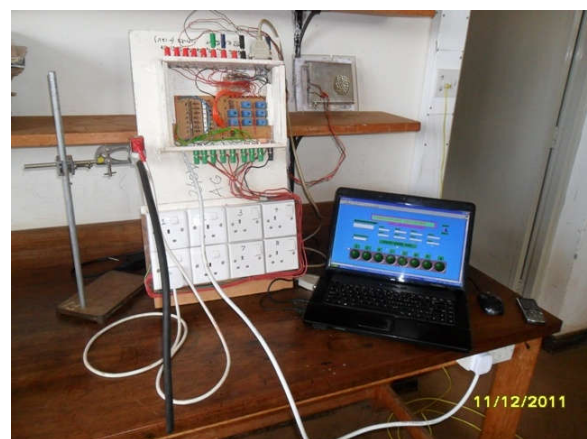
Fig. 9. Photograph for the designed firefighting system
