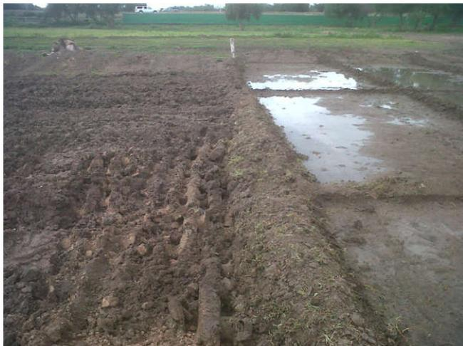
Figure 1. Expansive soils hydration by means of the “presaturation” method
