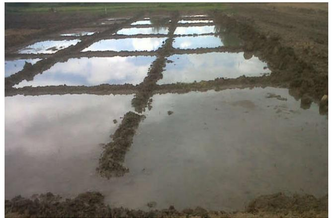
Figure 3. Expansive soil ponding by means of the “presaturation” method
