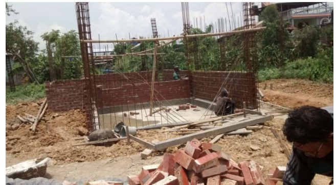
4. Upcoming wall of rain water harvesting tank
