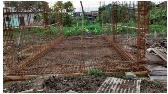
3. Preparation of the bed of the underground tank
