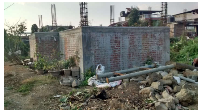
5. Two 15 ft by 14 ft tanks finished for terrace rain water harvesting
