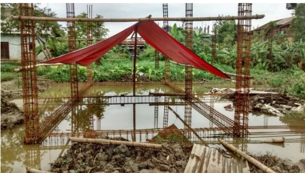
2. Preparation of the low lying ground as underground rain water harvesting tanks
