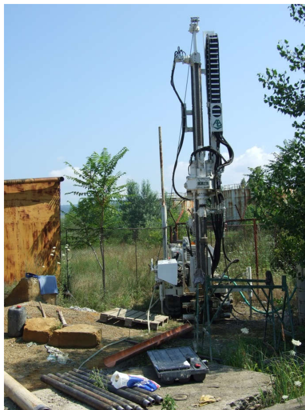
Figure 3. Drilling of borehole F1
