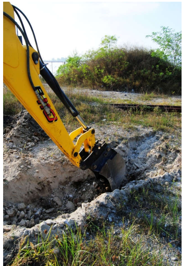
Figure 5. Digging of SP4
