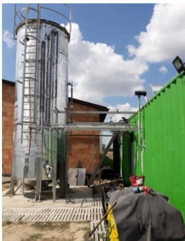
Fig. 4. Pilot installation - examples of techniques of the anaerobic fermentation of waste - mono-substrate reactor
