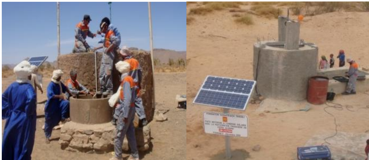
Figure 4. Solar pumping of the water in the southern Algeriaa
