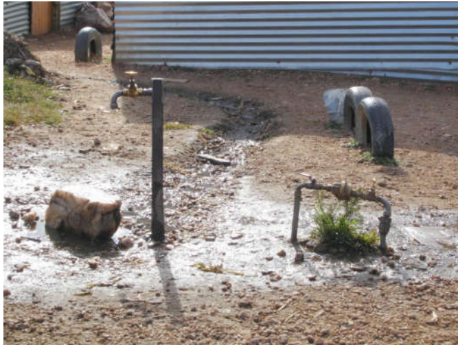
Fig. 1. Postpaid Standpipe and Meter
