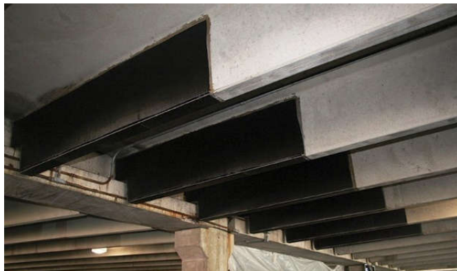
Fig. 1. FRP application on concrete beams
