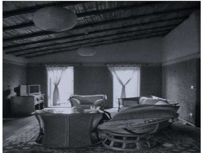
Figure 18. Flattened Bamboo used in roofing
