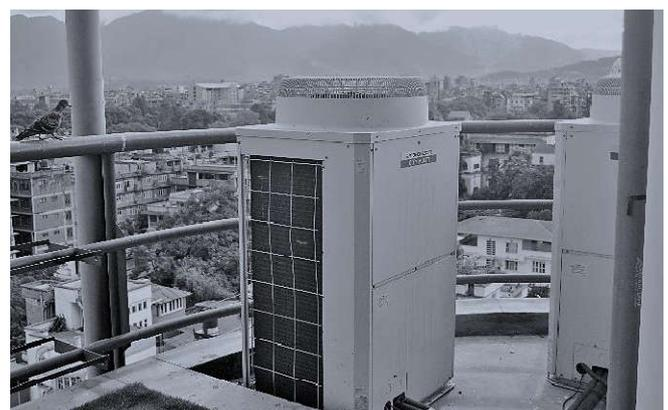
Figure 24. Outdoor Unit of VRV HVAC System
