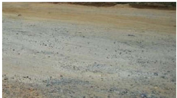
Figure 3. Existing Condition of road Due to Bad Drainage
