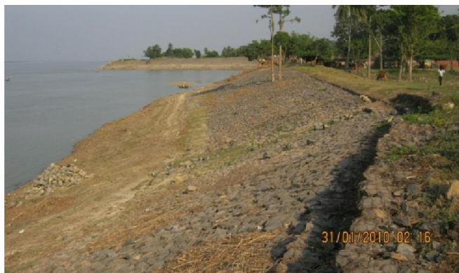
Plate VIII. Padma River bank protection through boulders with weir nets
