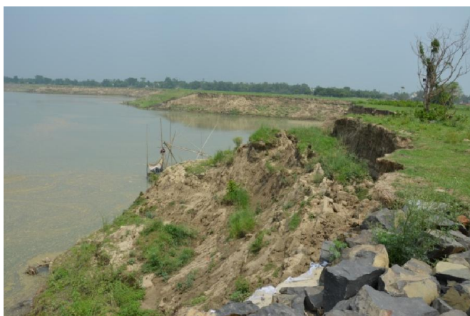
Plate IX. Bank protection by boulder washed away along Padma River bank at Maya (Lalgola)
